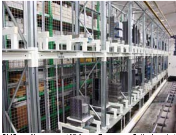
SMC utilizes a 167-foot Fastems Cell in their manufacturing processes. This Fastems cell is the longest in North America.
